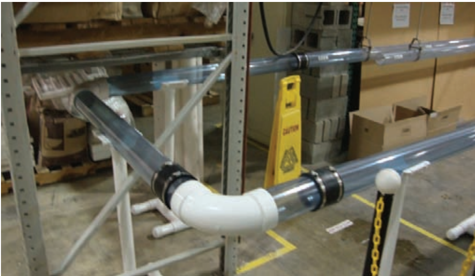
PHOTO 4-D VIEW OF 90° WIDE SWEEP BENDS
